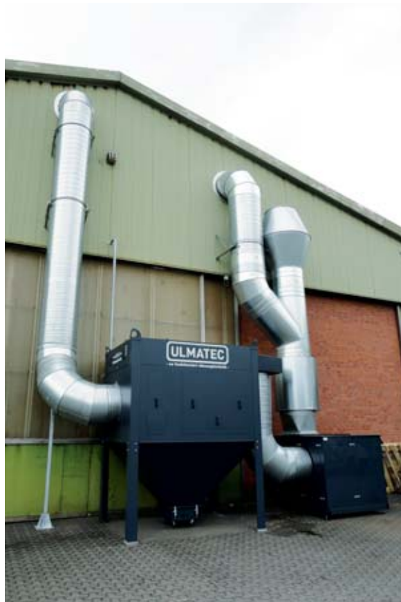
Filter unit FEP 320-16-8 with lateral condenser MRG 37 KW
