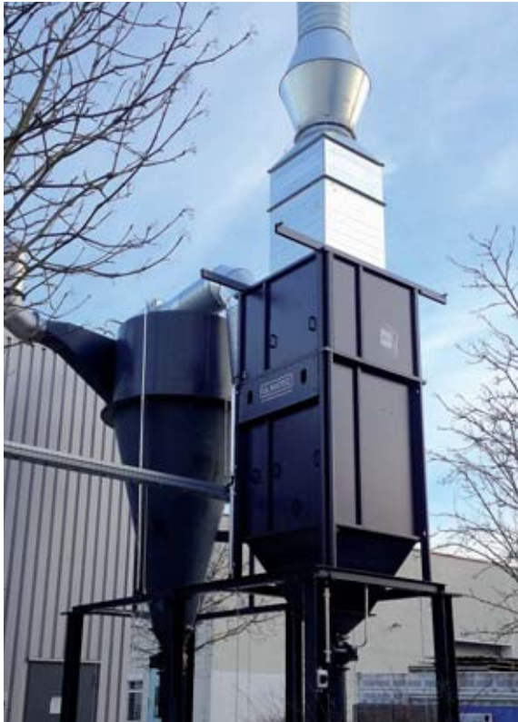
IES 25-49-6 / 15 MD with removal via cell wheel lock and cyclone pre-separator
