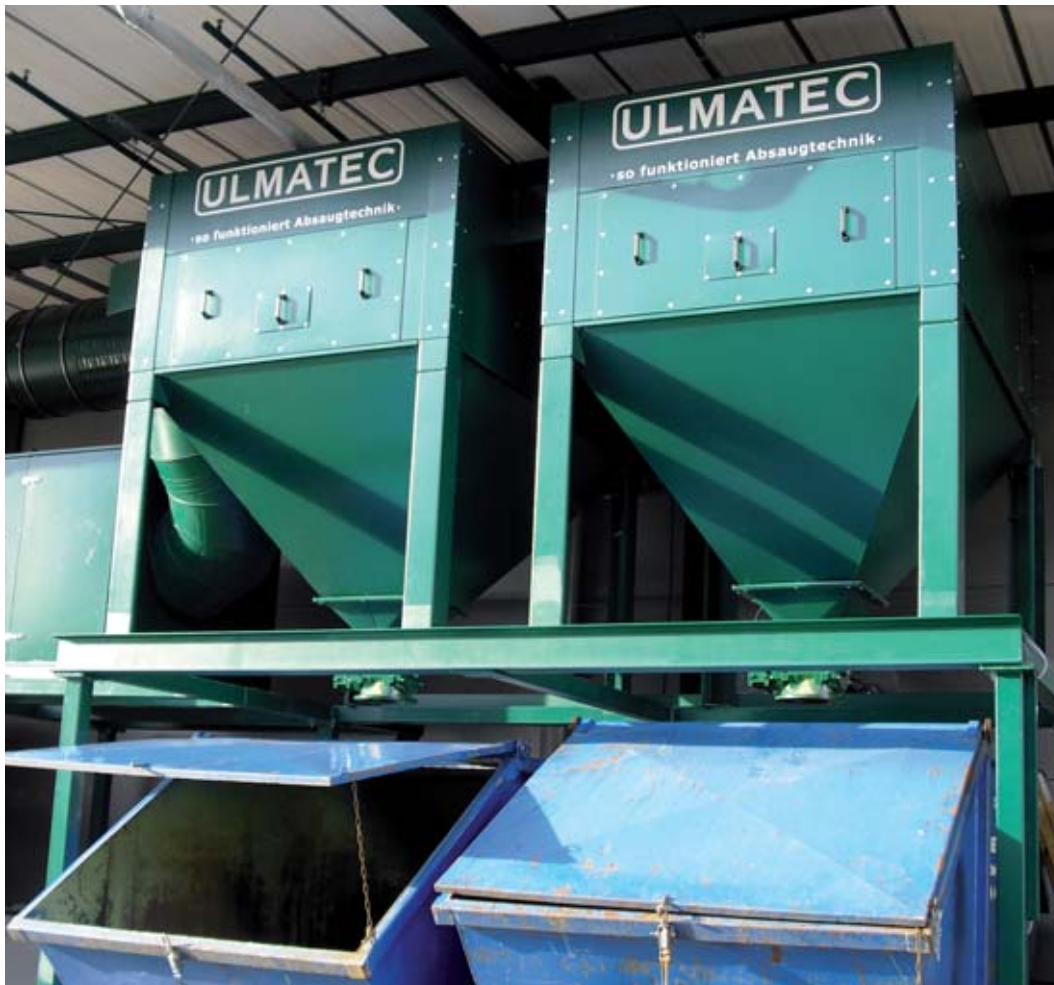
Filter unit FEP 320-32-8 (consisting of 2 x FEP 160-16-8)
