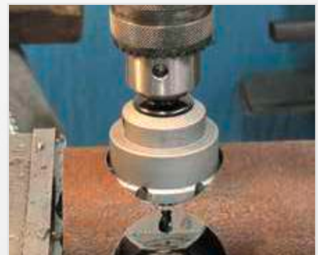
Drilling in pipes
